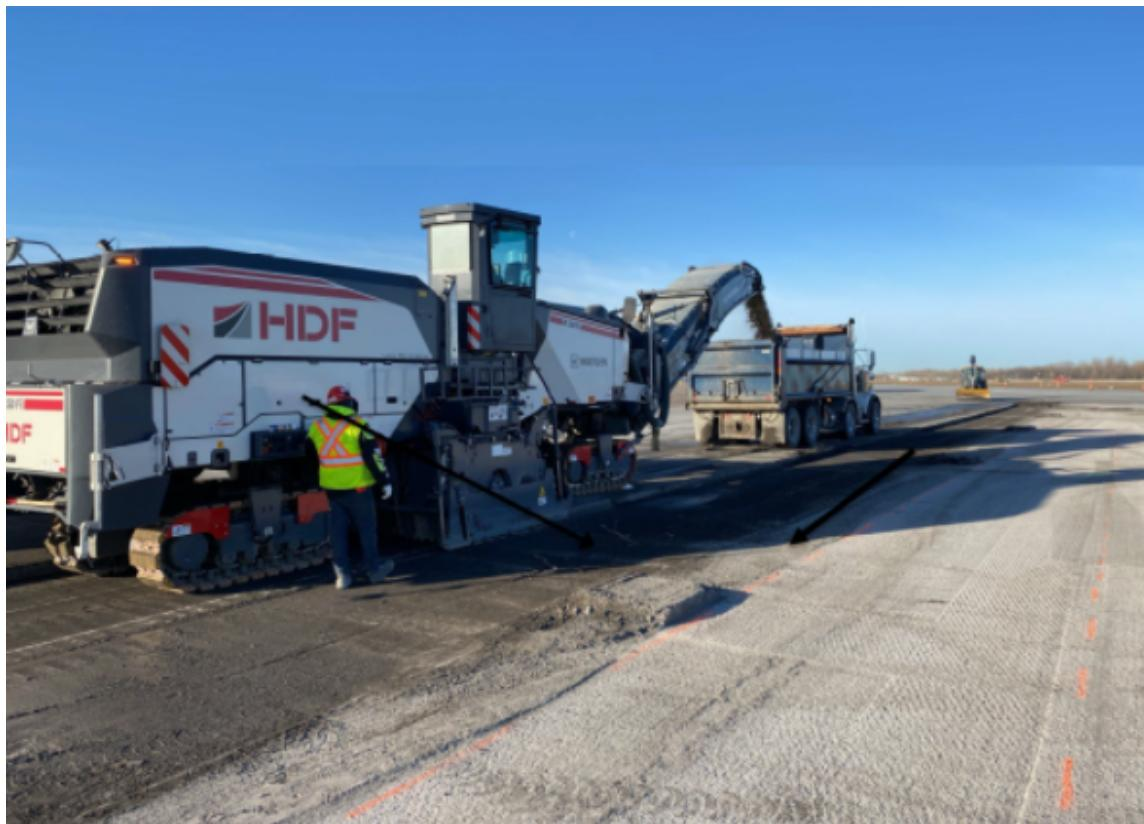
Leveling work above the concrete slabs on taxiway B3
