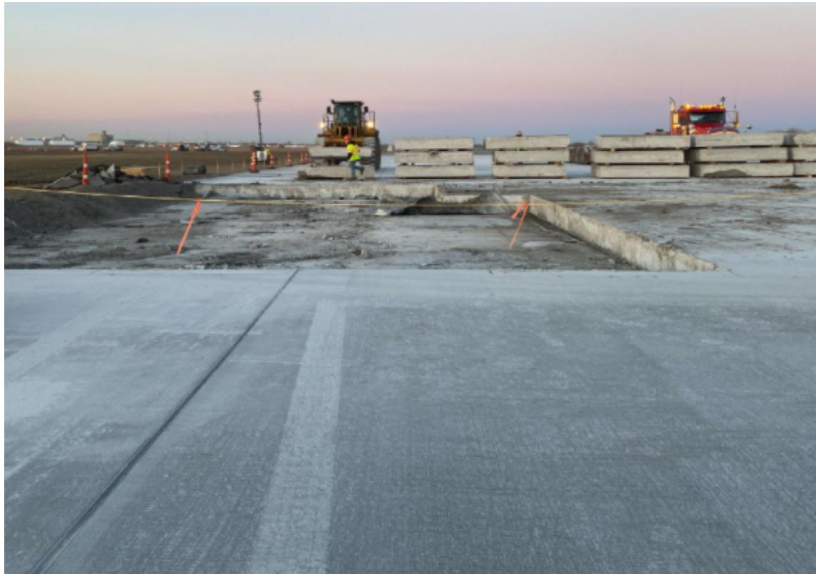
Removal of concrete transition slabs on the runway
