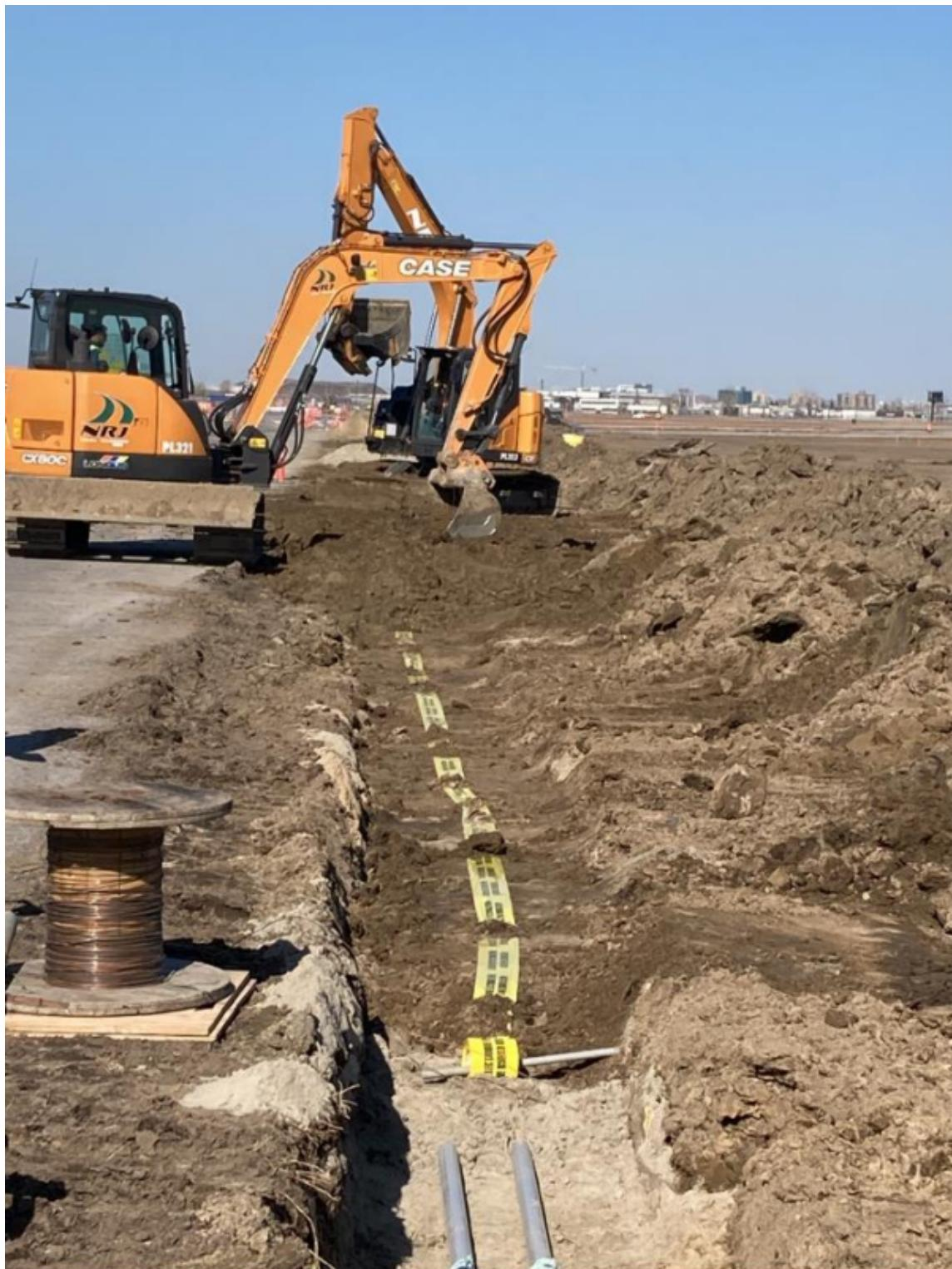
Installation and backfilling of new conduits on the edge of the runway
