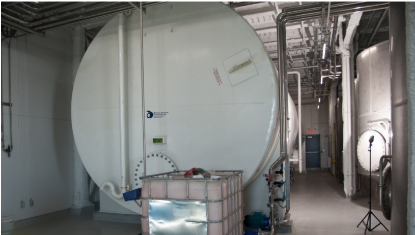
Step 5 The large white tank at left receives distilled product awaiting re-certification.
